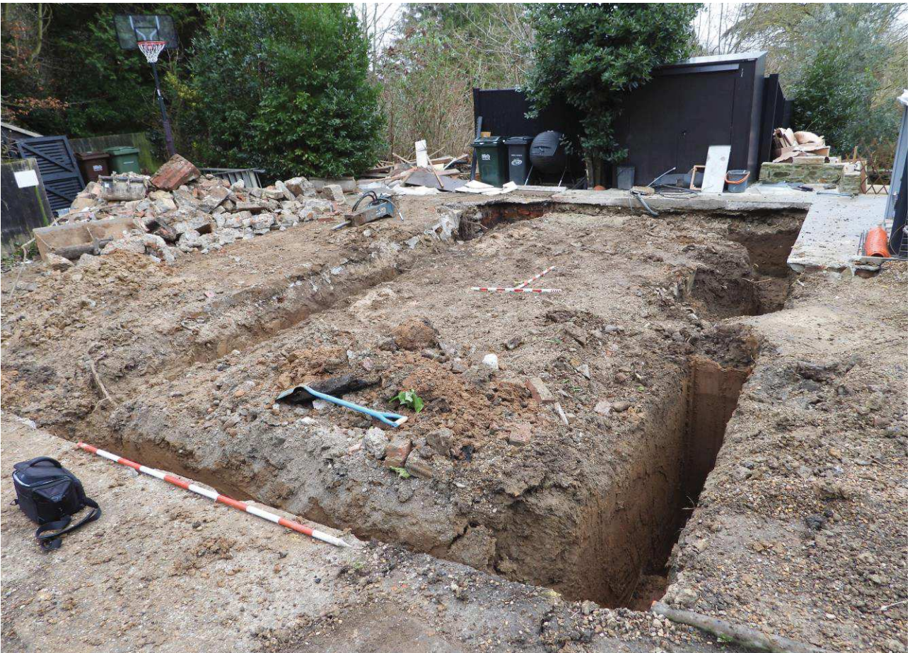
Plate 2: Foundation trench, looking southeast with two and two-one-metres scales.
